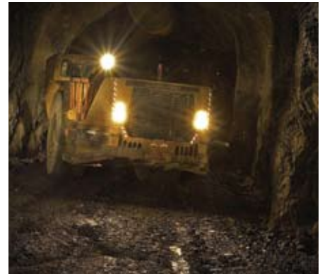
A typical unfinished underground road surface.
